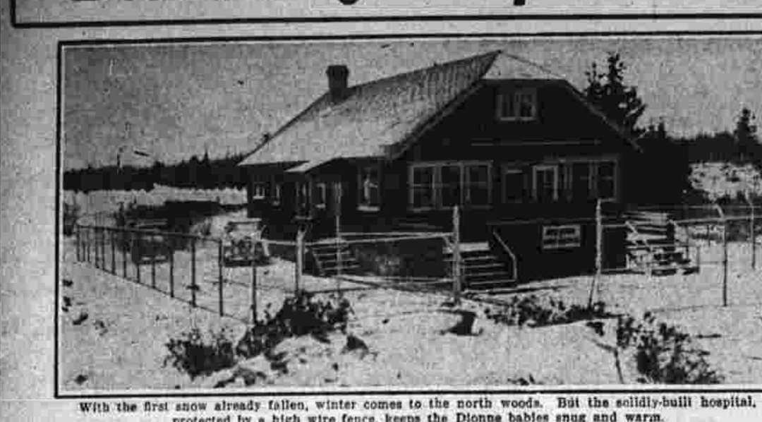
With the first snow already fallen, winter comes to the north woods. But the solid-bull hospital, protected by a high wire fence, keeps the Dionne babies snug and warm.
